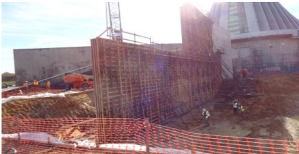
**While this work is in progress, new exhibit space interior concrete walls are being poured that will separate the new exhibit galleries and I -Max Theater. Once the old walls have been removed and the new galleries built, a new exterior wall and roof will be built over the exhibit space, the roof will be covered with soil and grass to match the other side of the museum.**
